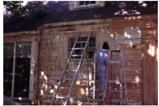
Use extreme care when stripping your house of paint. Chemical paint removers and lead in existing paint can be dangerous to humans and heat removal may result in a fire.
