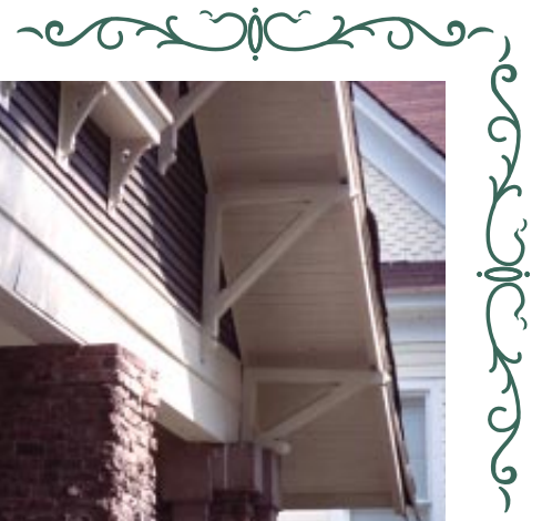
Deep eaves with wood brackets are an essential element for a bungalow house.
