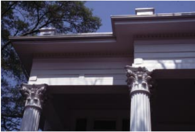
This photograph is a good example of a typical classical cornice.
