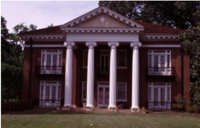
A central portico supports a pediment with large modillion blocks in this example of the neo-classical style.
