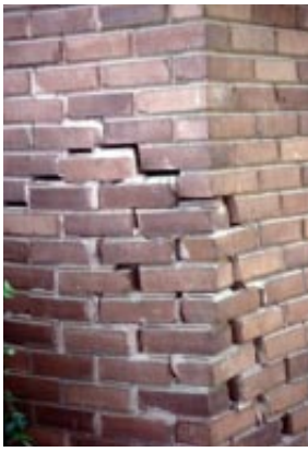
Water penetration and building settlement may cause damage to brick.
