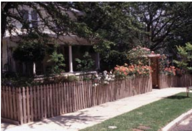
This simple board fence is complemented with landscaping and a central entry element. The pressured-treated wood should be painted after it ages a season.
