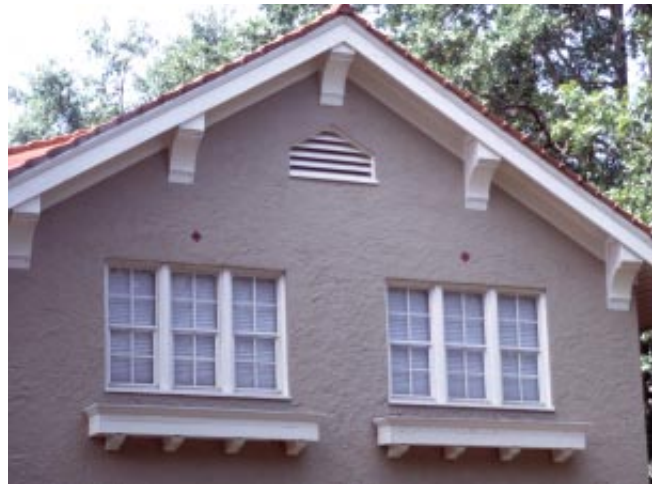
These multiple double-hung windows have no exterior trim because they are placed in a stuccoed wall.
