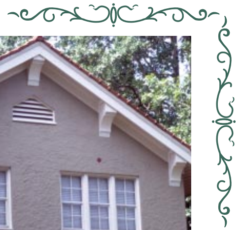
These multiple double-hung windows have no exterior trim because they are placed in a stuccoed wall.
