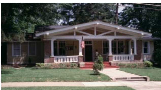
The low, horizontal lines of this house are typical of the Bungalow style and the exposed structural rafters are the trademark of the Craftsman movement.
