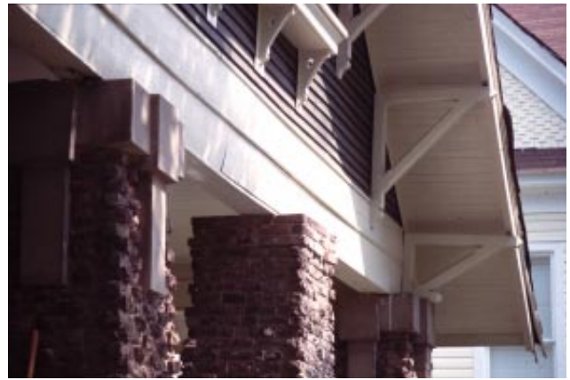
Deep eaves with wood brackets are an essential element for a bungalow house.
