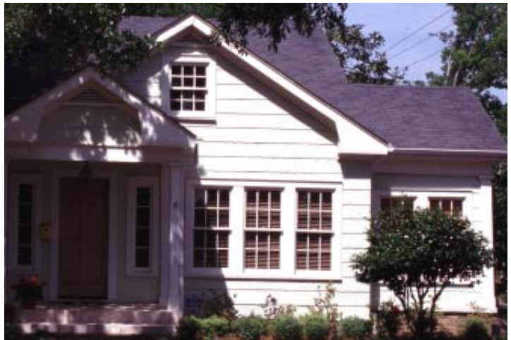
Earlier examples of synthetic siding include asbestos shingles as seen here.
