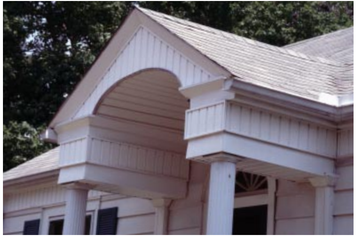
The use of synthetic siding on this portico hides any detailing that might enhance the entry.
